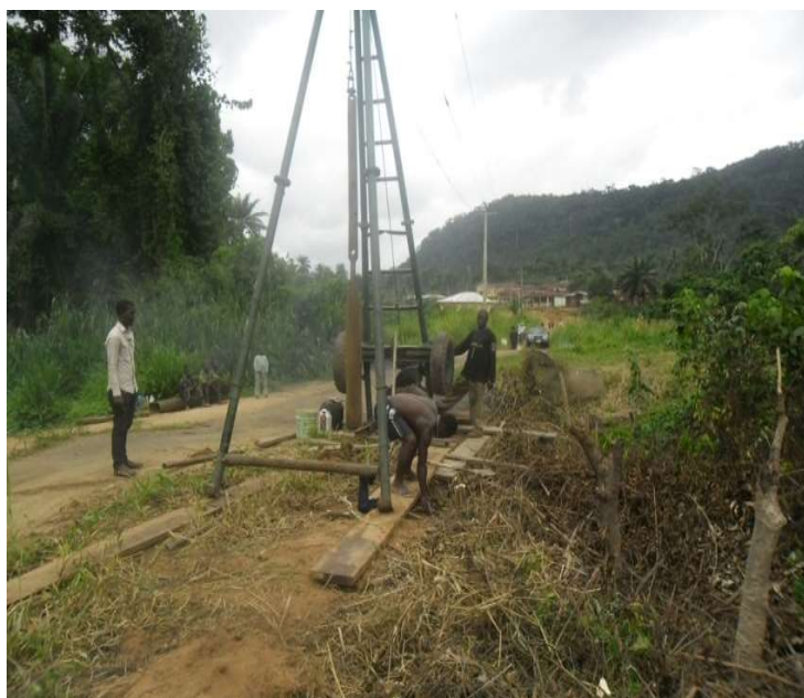
Eti-Oni Bridge Site Deep Soil Investigation: Boring of Probe points at the Design stage.)
