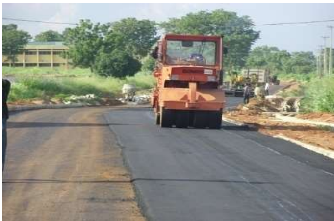
Asphalt Roller Compacting on the laid Asphalt at KM 0+600
