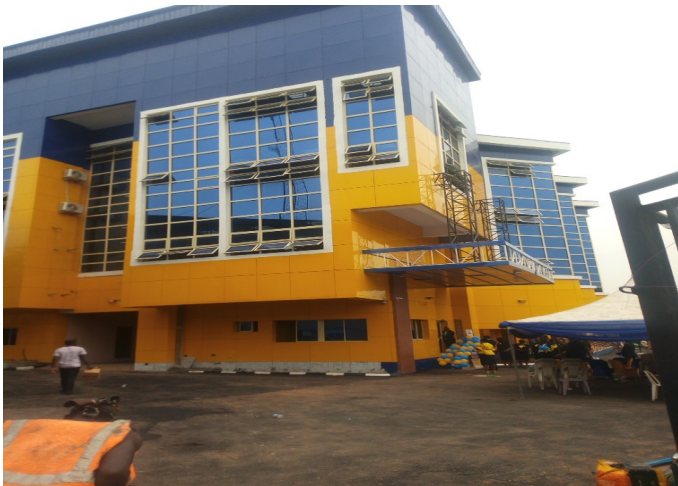
Construction of 3-Storeys Human Resources Management Building WAEC, Yaba Lagos
