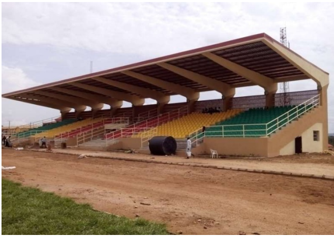
1000 Seat Capacity Stadium, Adeyemi College of Education, TETFUND Project.
