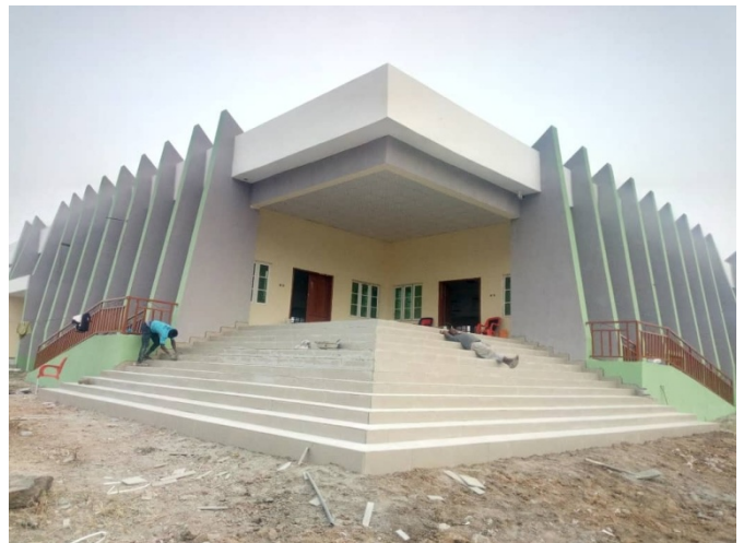
Construction of Twin 200 Seat Lecture Theater, Federal College of Education, Okene, Kogi State
