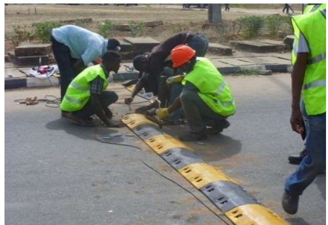
Rubber Bump Installation, Along University Main Road, University of Ilorin
