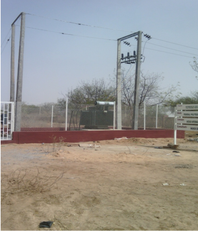
Extension of 33KV Line, Federal Polytechnic, Damaturu, Yobe State
