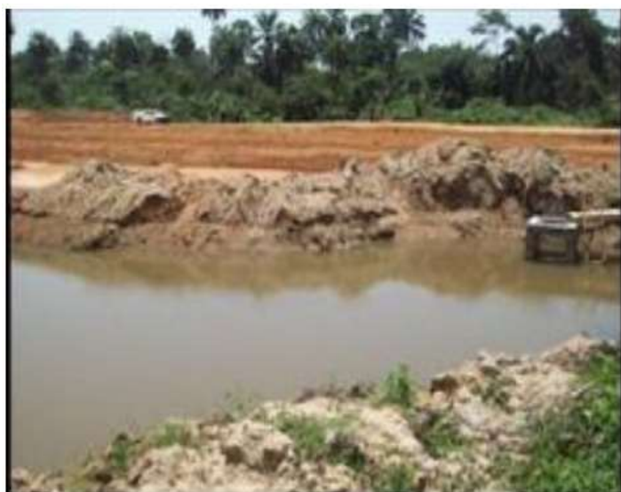
Plate 1: Iragbiji Earth Dam Site, Osun State
