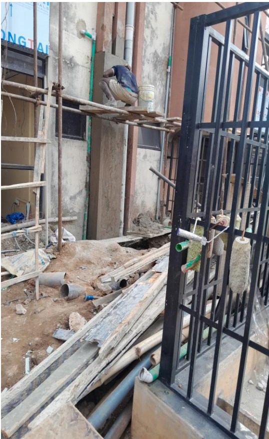
Jacketed Column on the 5-storey JAMB Building at Ogba, Ikeja, Lagos
