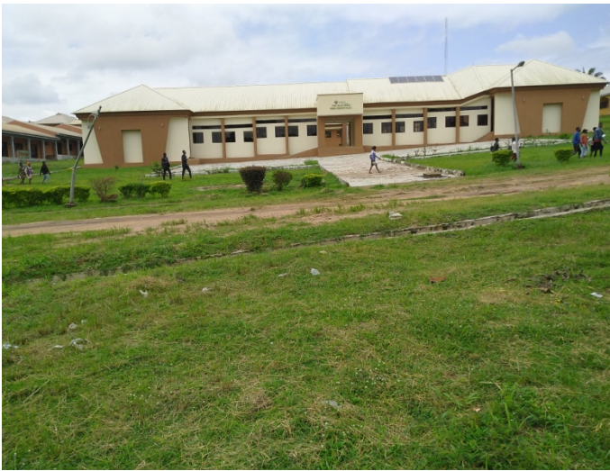
Completed 6 Block of Classrooms at Adeyemi College of Education
