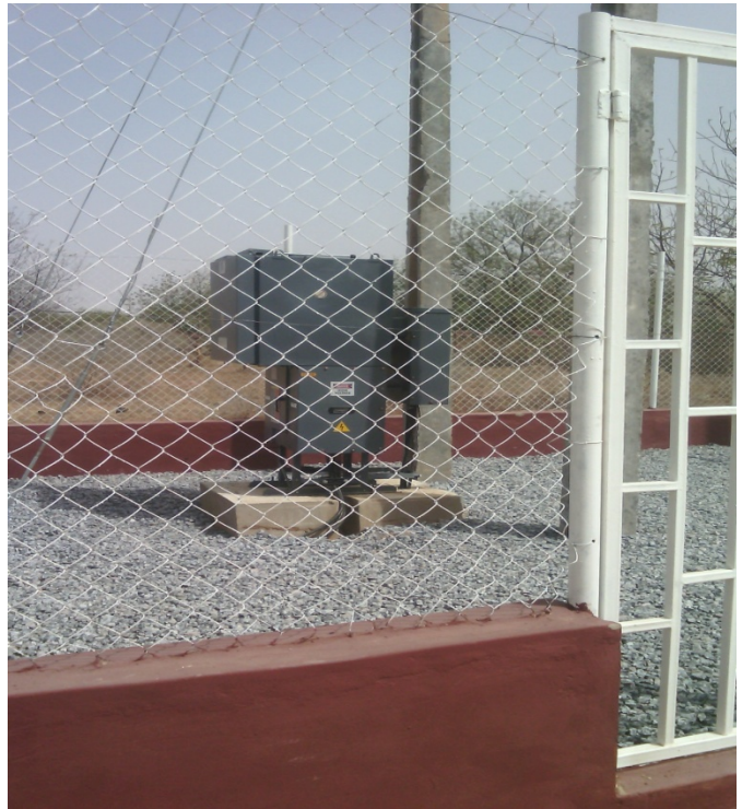
Installation Of 1No. 500KVA Perkins Generator and Accessories, Federal Polytechnic, Damaturu, Yobe State
