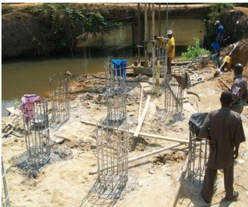
Pilling Operation On Eti Oni River Bridge Along Ilesha-Ipetu Ijesha Road, Osun State.
