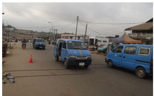
Laying Of Rock Boulders As Subsoil Drainage Carpet For The Road Pavement
