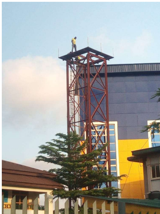
Over Head Tank Construction for WAEC Office, Yaba Lagos State
