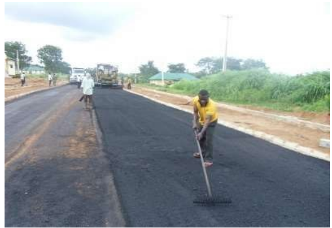
Asphalt Overlay, Along Bank Trunil Hostel Road
