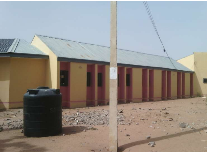
Renovation of Student Hostel, Federal Polytechnic, Damaturu, Yobe State
